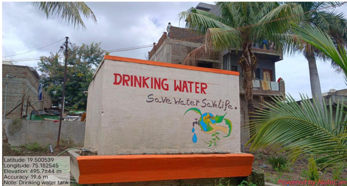
Drinking Water tank Near the Botanical Garden
